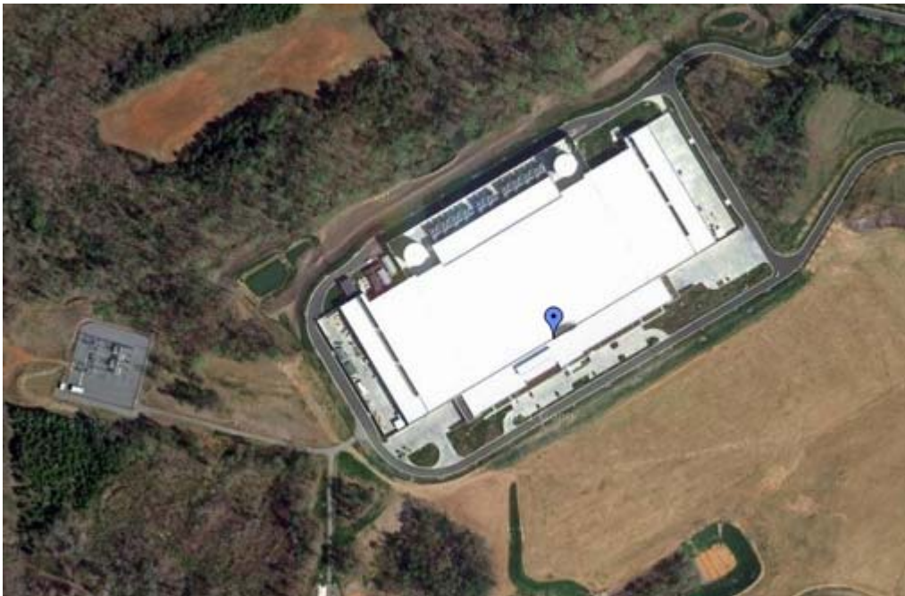
New Apple data center in Maiden, N.C. (Image: GoogleEarth)
